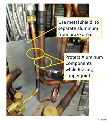
Fig. 33 – Use Braze Shield to Protect Aluminum
