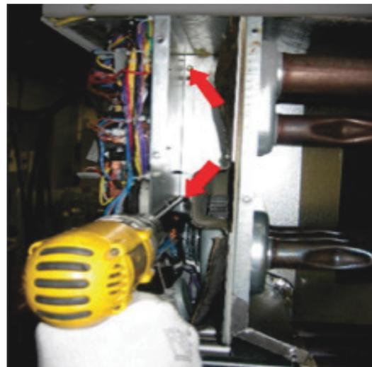
**Fig. 33 – Removing Screws Behind Heat Shield** <sup>A210077</sup>
