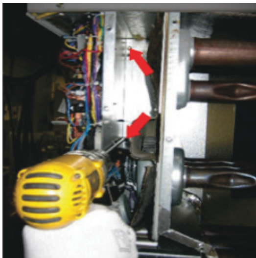
Fig. 32 – Removing Screws Behind Heat Shield
