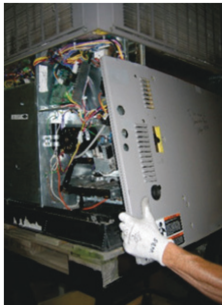
Fig. 36 – Replacing Right Side Panel
