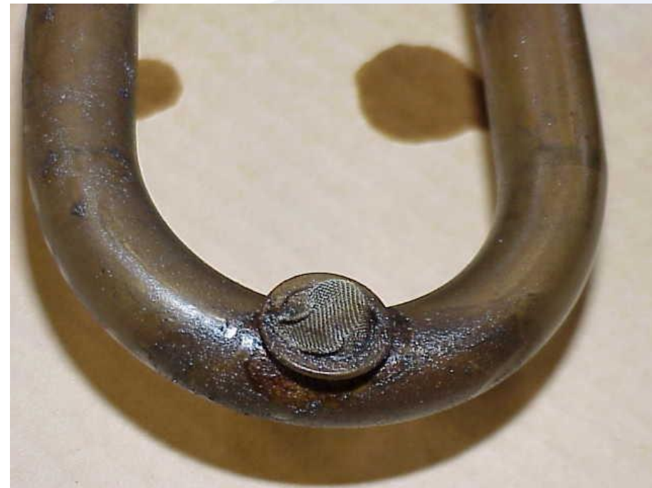
Screen damage and corrosion
